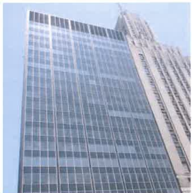
Tishman Building Currently being considered for mixed-use development opportunities.
